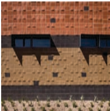
Concrete masonry units in varying colors and textures
