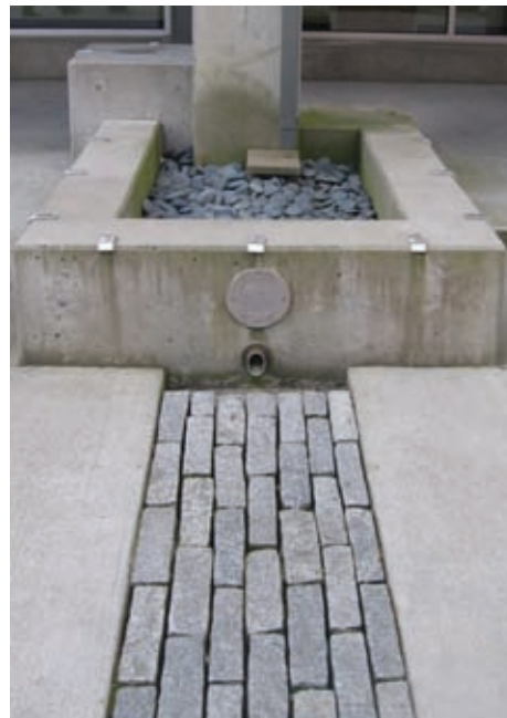
(upper) Water from disconnected roof leader enters pervious surface and filters water before discharge to porous pavement.
