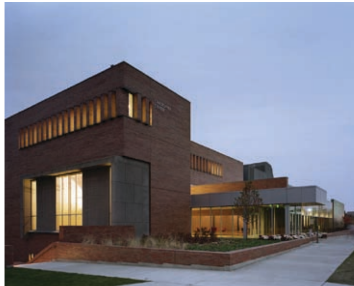
(left) A protruding canopy marks the building entry and provides weather protection.
