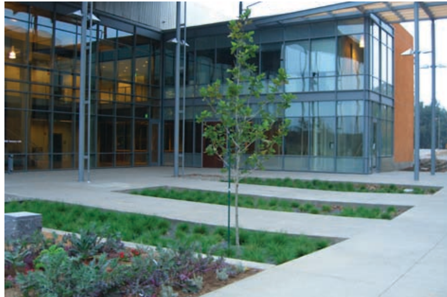
(lower) Stormwater planters provide areas for excess water to collect, filter and infiltrate.
