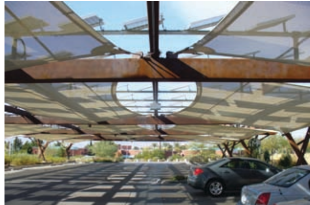
(upper) Shade structure with photovoltaic panels provide shade for cars and collect energy for use.
