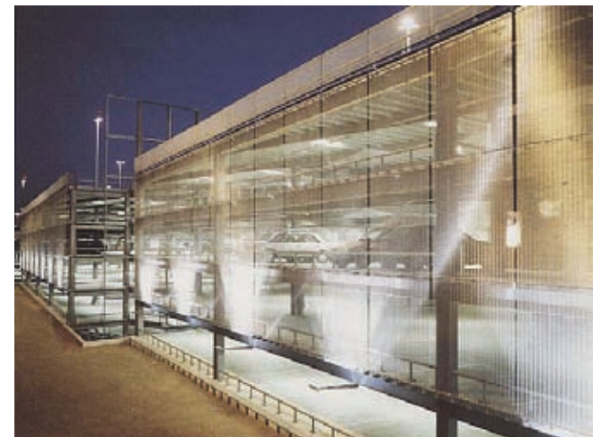
(below, all) Parking structures should be articulated with form or texture to temper visual impact.
