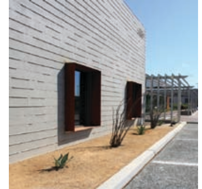
Cast-in-place concrete with weathering steel accent at window boxes
